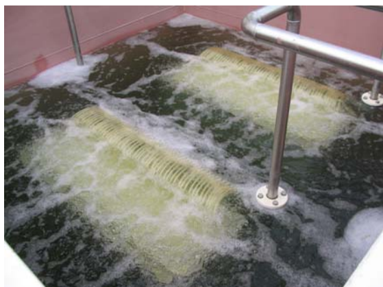
Fig 2.- Detail of the membrane reactor.
