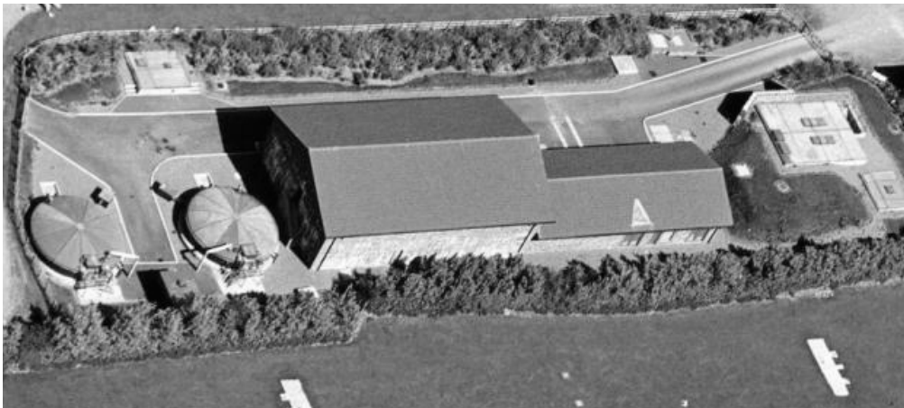
Figure 1: The Porlock MBR treatment plant
