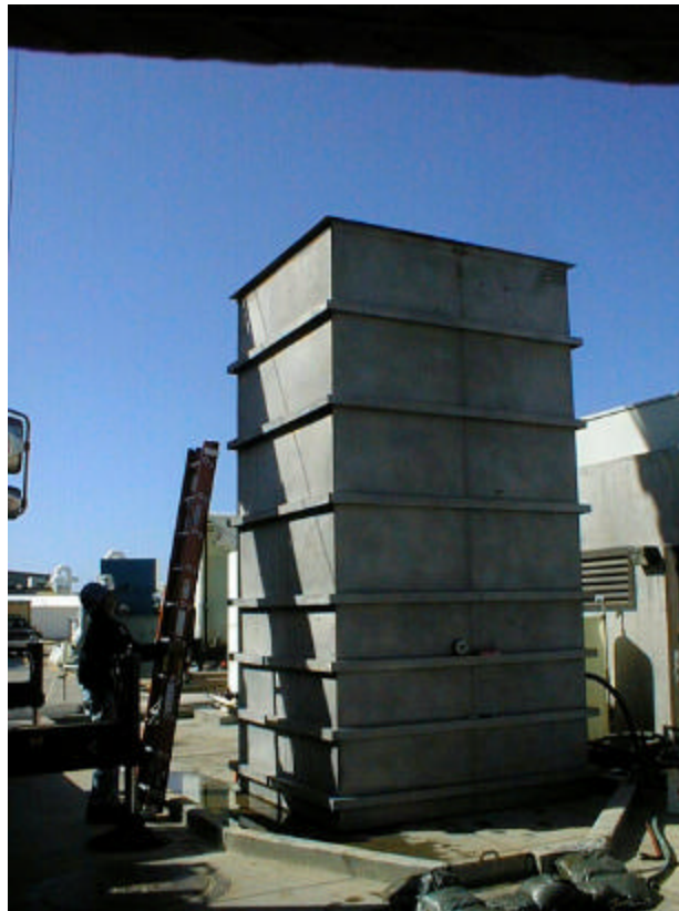
Figure 2-1 Photograph of the Kubota MBR Pilot Process Tank
